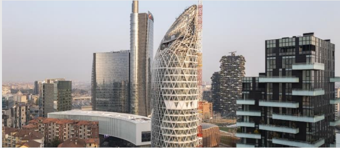
Torre Unipol, Milano
